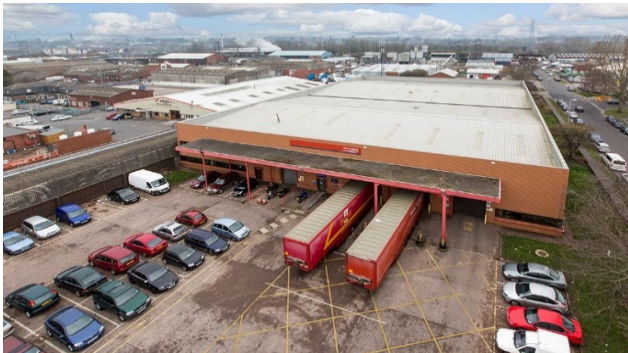
Exeter, 13 Trusham Road, Marsh Barton Industrial Estate
