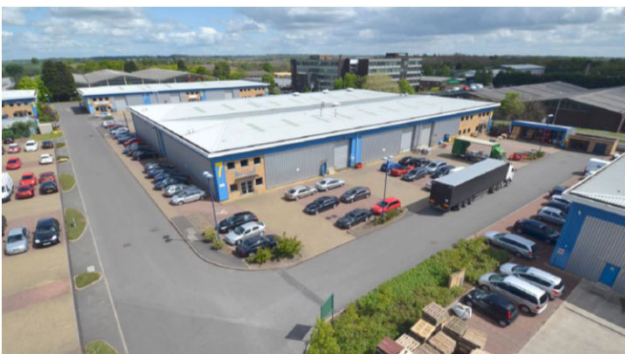
Northampton, IO Centre, Lodge Farm Industrial Estate
