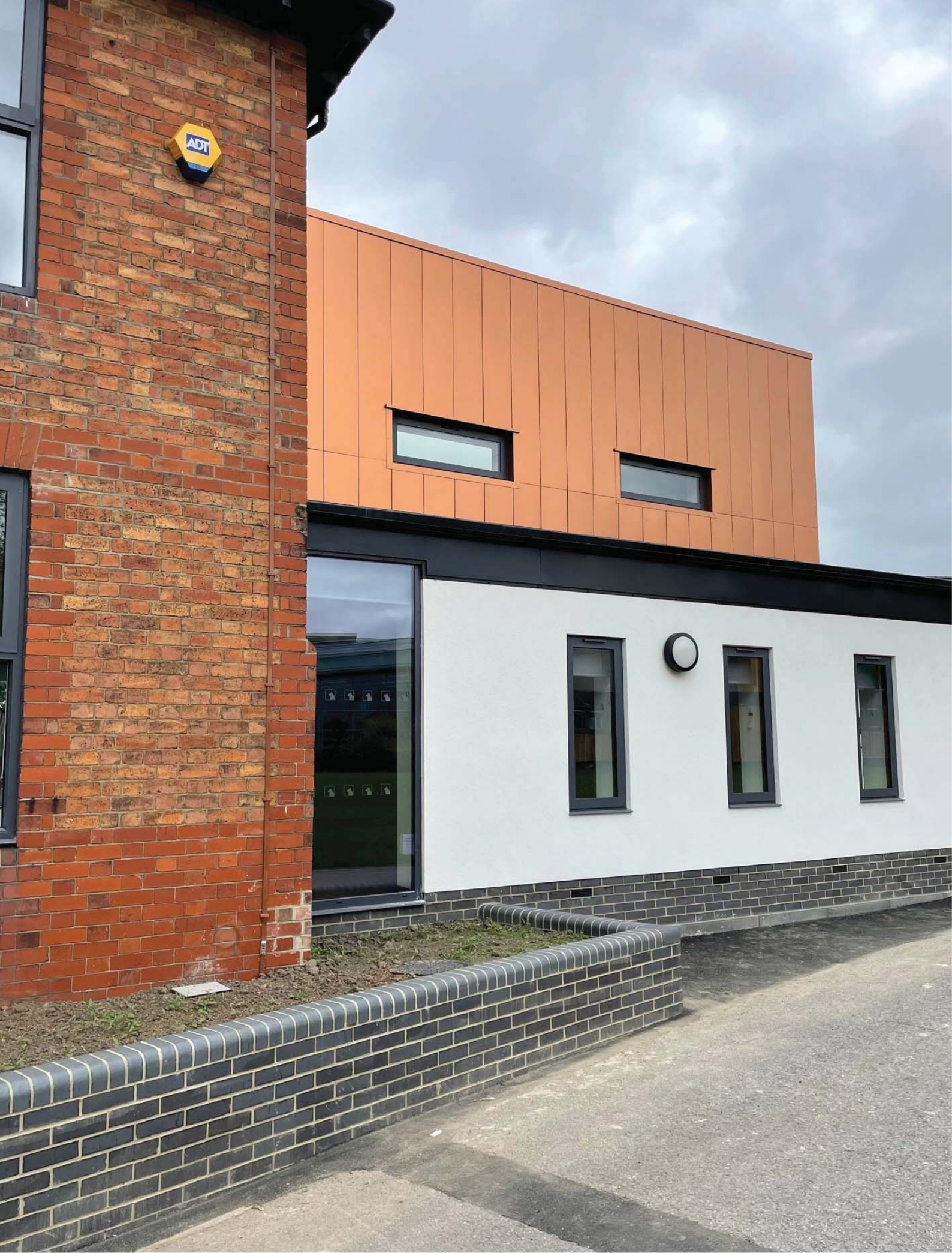
System Roofing Services Ltd - Dead Dog Gallery, Sixth Form College, Durham
