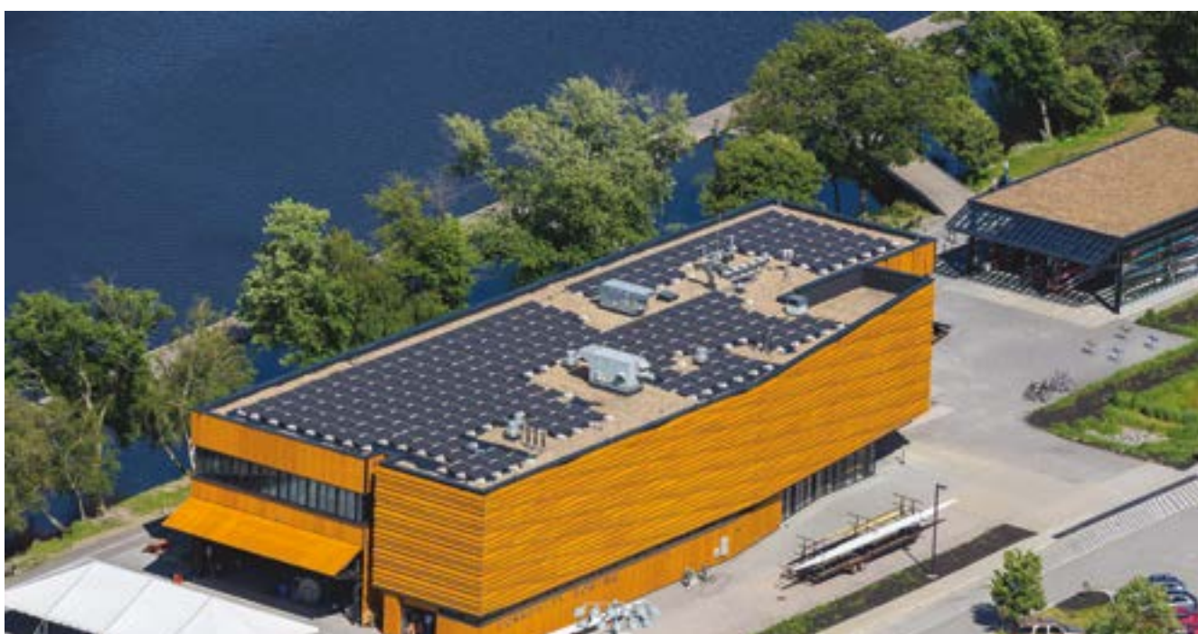
Rooftop solar system at a community rowing facility in Massachusetts, part of SED Solar Portfolio
