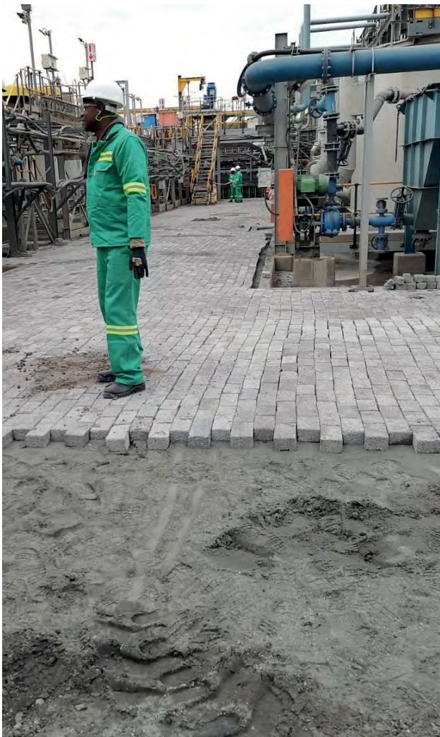
South Africa_Bricks from brick making project used at Inyoni plant.
