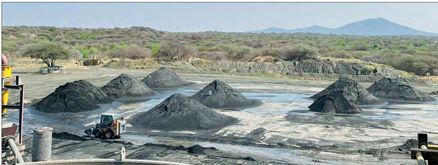
South Africa_Thutse Plant.
