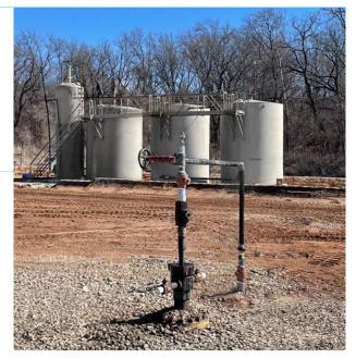
Permanent production facilities have been installed, comprising oil storage tanks, separator and flowlines and light crude oil with an API of 32 degrees is being sold. To date, over 3,000 barrels of oil have been produced and sold whilst testing.
