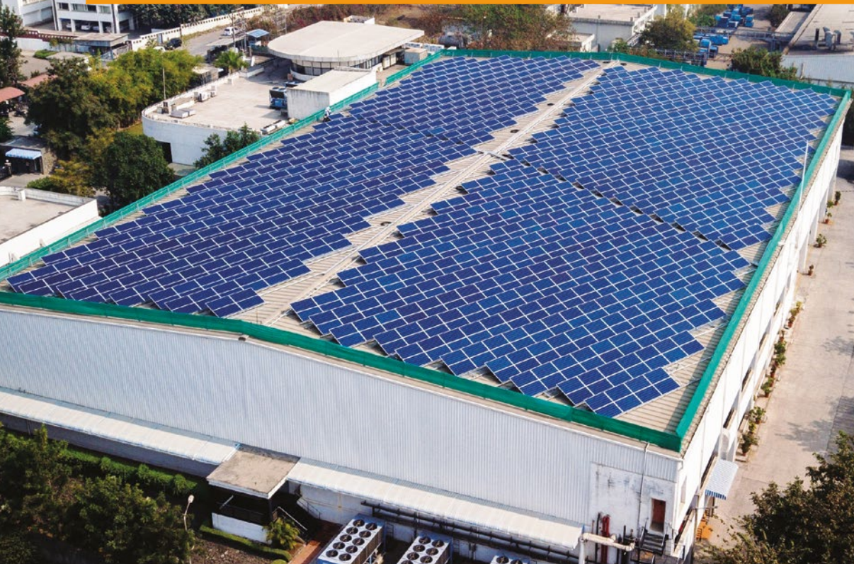
◀ Solar panels at our manufacturing facility in Pune, India.
