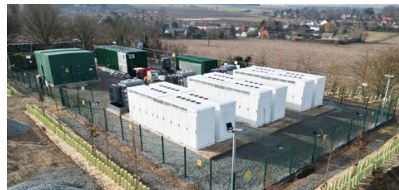
The Company's 11 MW / 22 MWh Broadditch project was successfully energised in March 2023. Broadditch, located in Kent, was the Company's second project to be energised.
