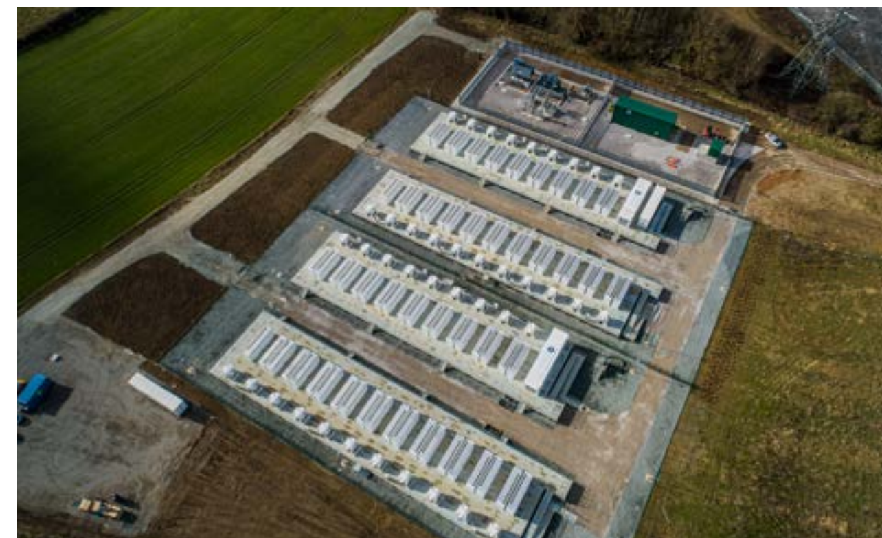
Aerial view of the Company's Pillswood site, Europe's largest BESS by energy capacity (98 MW / 196 MWh).
