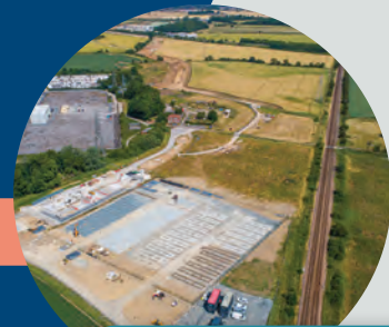
An aerial view of the 196 MWh / 98 MW Pillswood BESS prior to construction.
