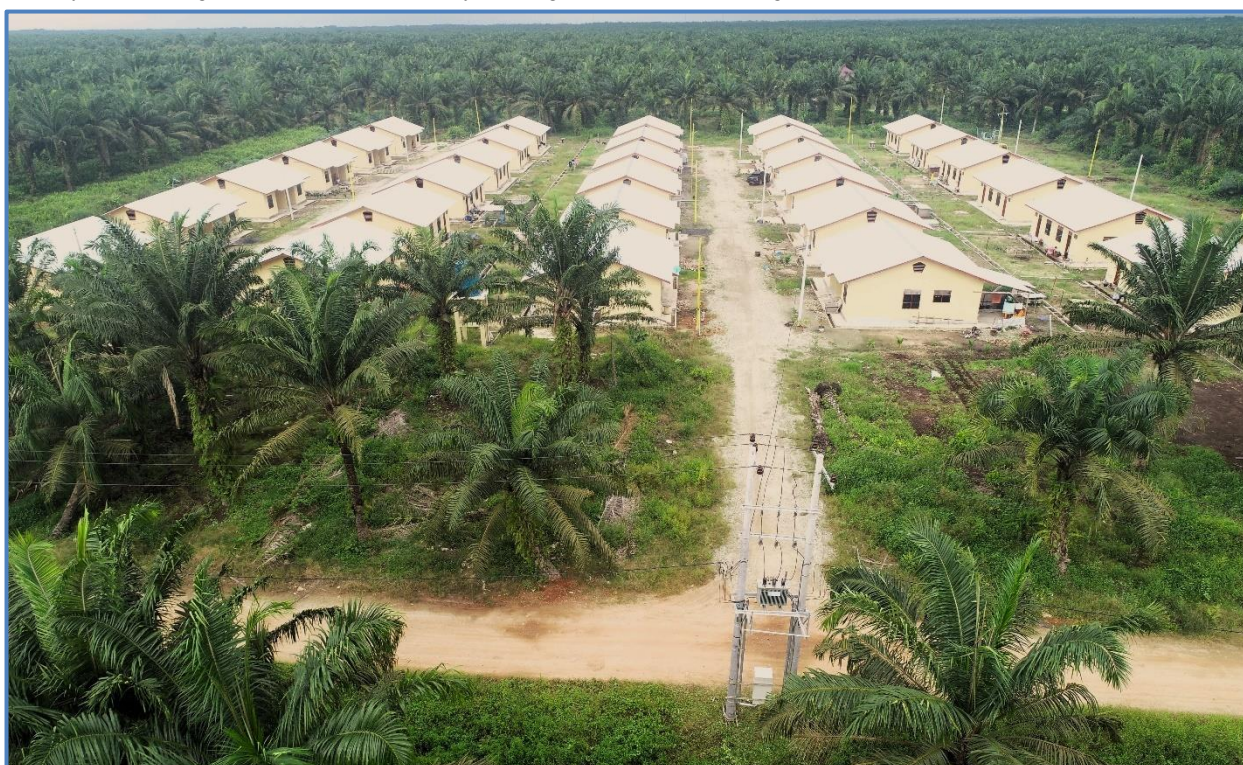
Electrification of workers housing in HPP
