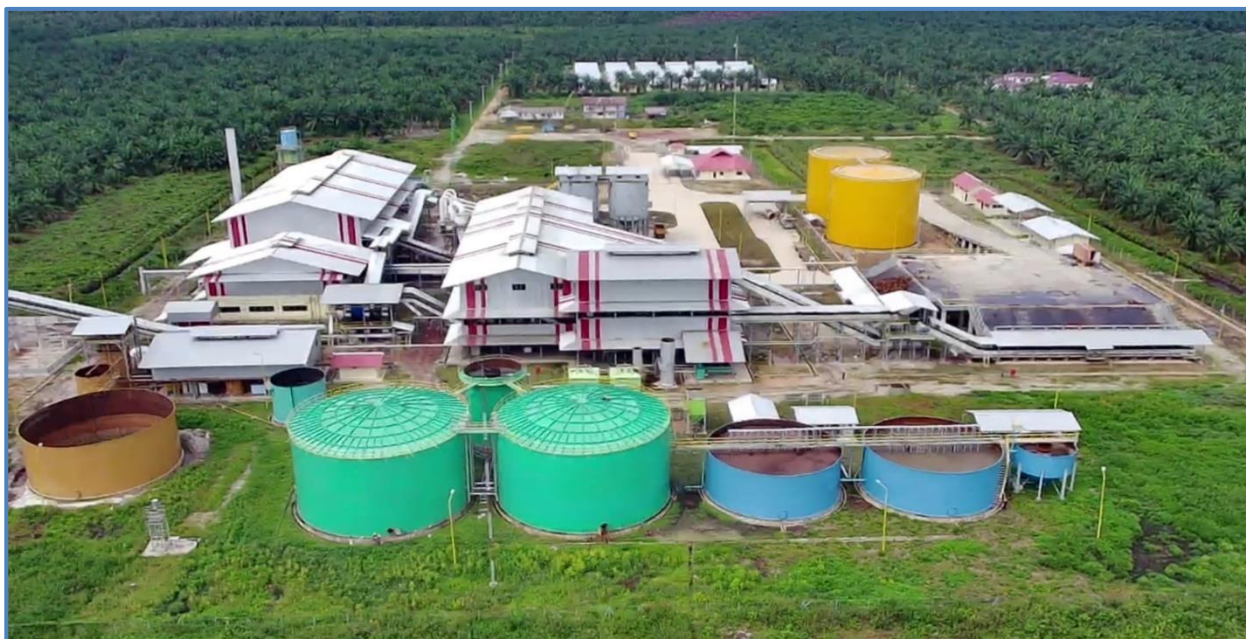
HPP Mill finally completed
