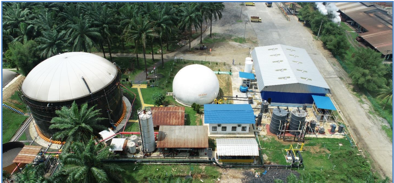
Newly built BioCNG Plant in Blankahan
