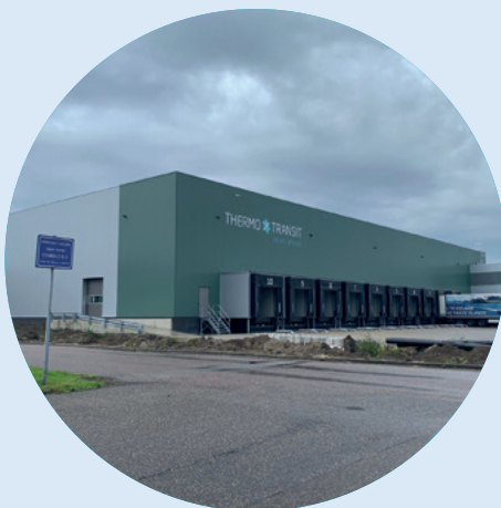
Extension project, Waddinxveen, Netherlands
