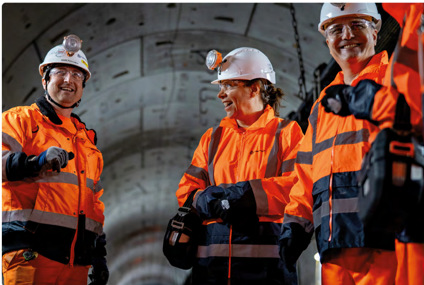
At the Woodsmith project's Lockwood Beck site, non-executive directors Magali Anderson (centre) and Marcelo Bastos (right) are shown around the Mineral Transport System (MTS) tunnel by tunnel area manager Mark Pooleman.
