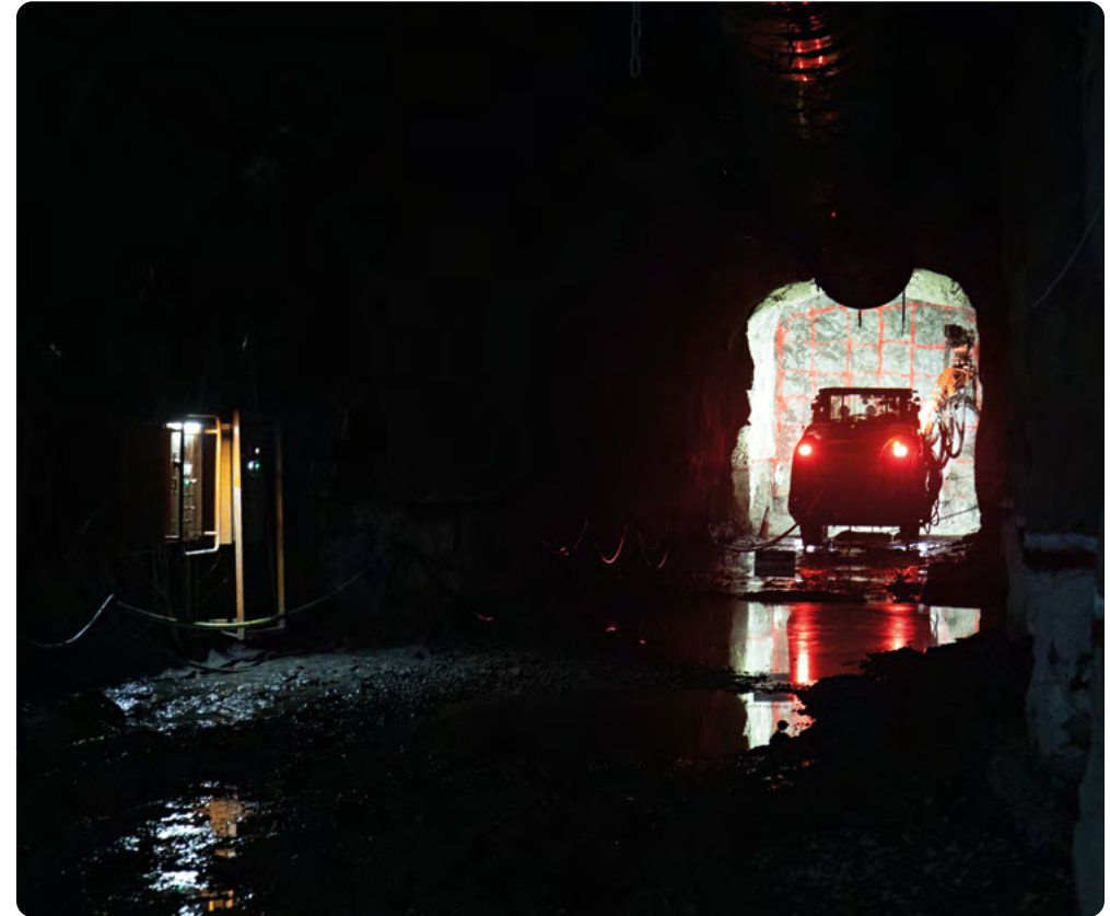
Venetia, South Africa's premier diamond mine, is transitioning from open pit to underground mining. Clearly visible in front of the drill rig is the high-tensile steel mesh that is applied, ahead of drilling, on stope roofs and walls to protect operators in the development area.
