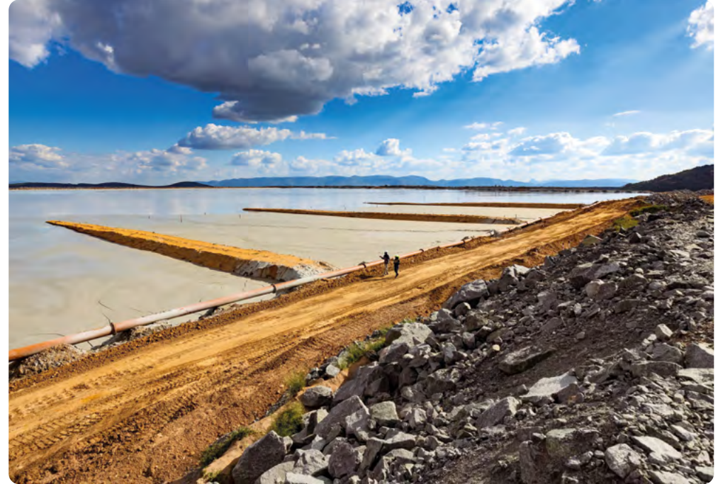
Mogalakwena PGMs mine in South Africa is piloting the first brownfield application of hydraulic dewatered stacking (HDS) tailings at Anglo American.
