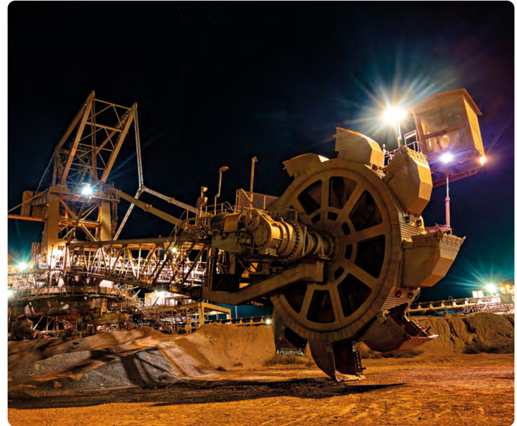
At Kolomela, this bucket wheel excavator and stacker reclaimer work in combination 24/7 to reclaim iron ore and then stack it in bulk quantities.
