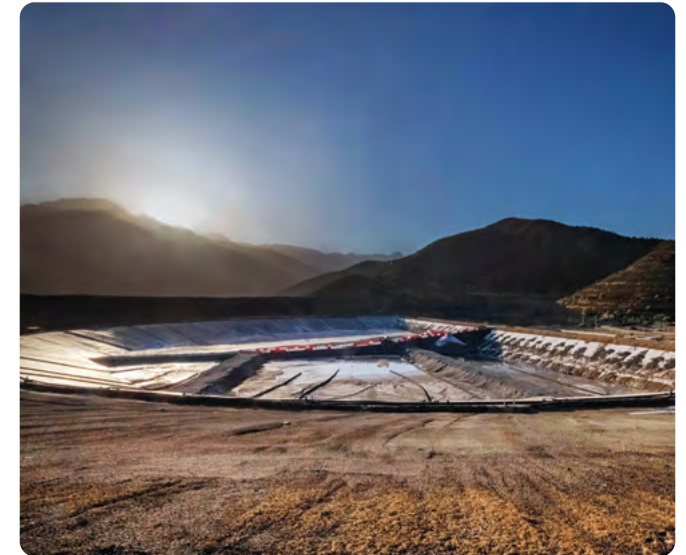
Neatly landscaped hydraulic dewatered stacking (HDS) tailings at El Soldado. The tailings are able to be remediated into dry and economically viable land following the mine’s closure.
