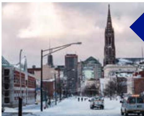
National Grid emergency crews work in Buffalo, New York, on 25 December 2022.
