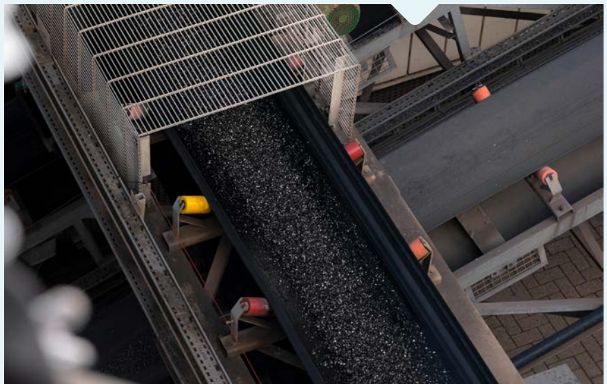
Gravel, sorting line, ATM Moerdijk
