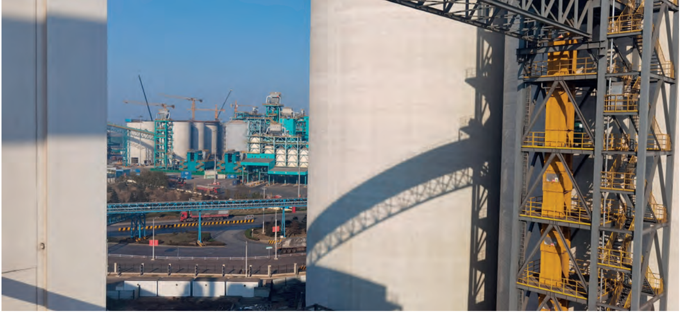
Aerial view of crushing plant and elevator equipment in Quindao, China.
