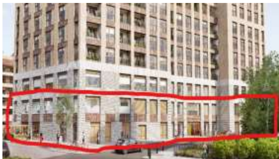
Peel Precinct Health Centre, South Kilburn
