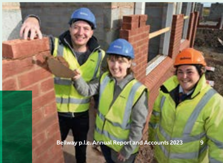
↓ Couple laying a brick in their new home with Assistant Site Manager Maddie Dale.
