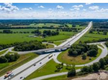
The A7 Motorway project is an availability-based design, build, finance, operate and maintain project located between the cities of Neumünster and Hamburg in Germany. The project comprises c. 65 km of highway widening from four to six lanes including 11 interchanges, six parking facilities, four rest areas and 79 engineering structures including a 550 m noise tunnel at the City of Schnelsen.
