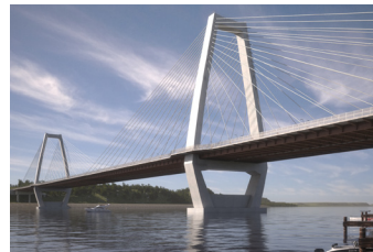
Ohio River Bridges US
