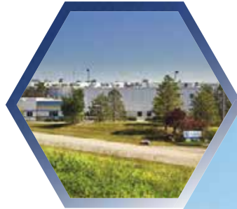
Foam manufacturing facility, Kentucky, USA
