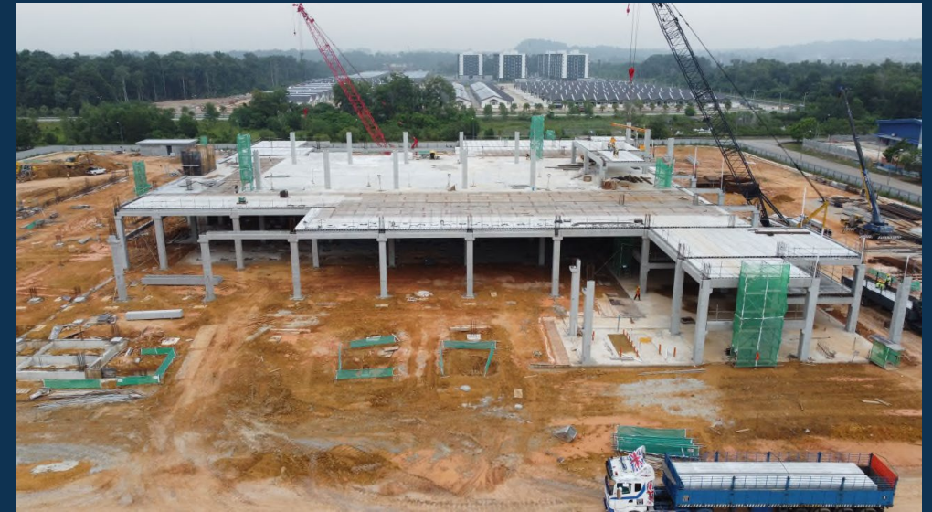
Construction progress at our site in Malaysia (July 2023)
