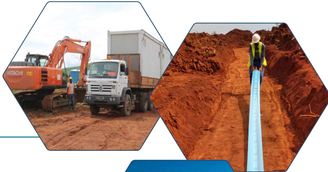
Ongoing earthworks and civil construction programs at the Longonjo Project
