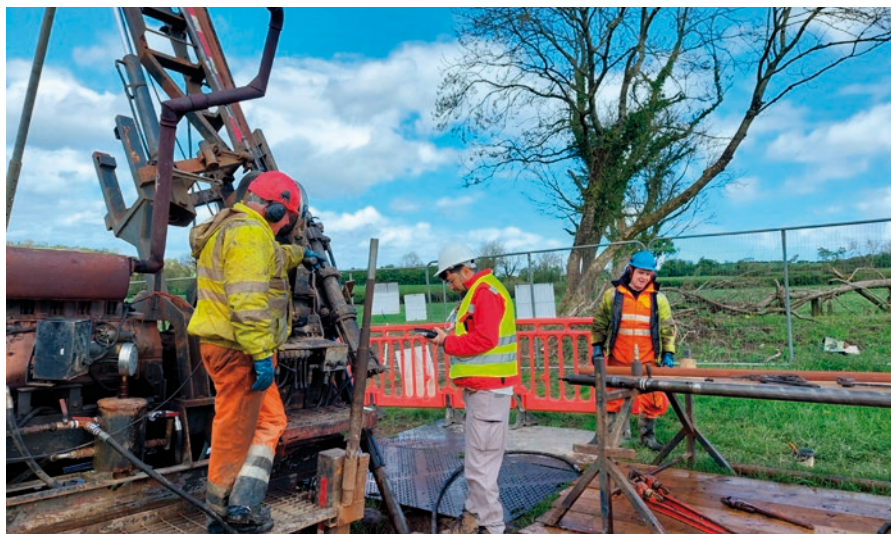
Drill Rig being set up on site at Clontibret Gold Deposit
