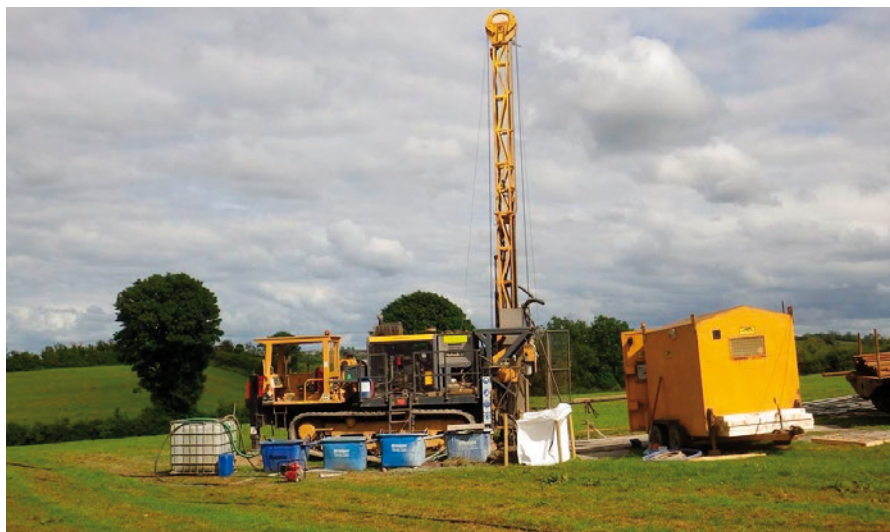
Drilling on Clay Lake Gold Target
