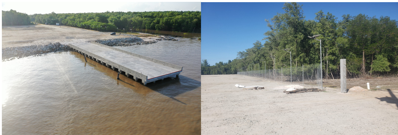
Images: Trestle / Fence installation
