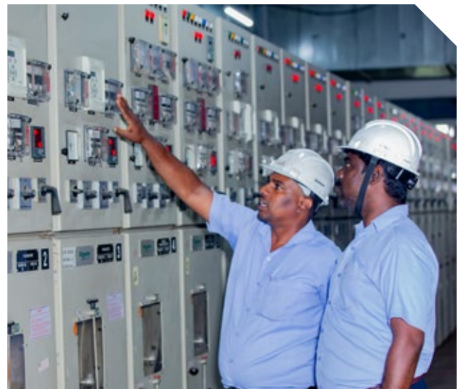
▲ Inspection work on relay panel
