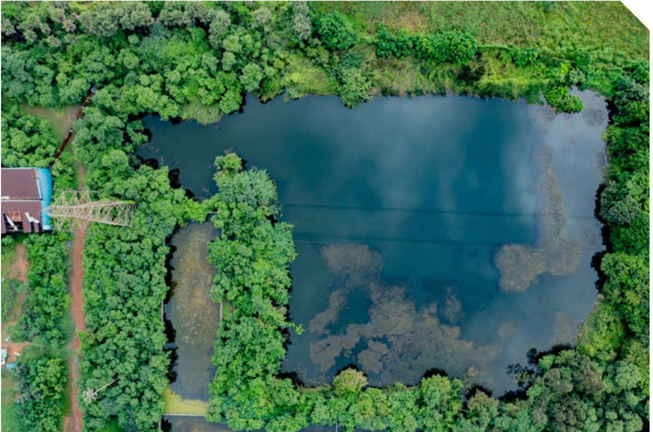
▲ Bird's eye view of the rainwater storage pond
