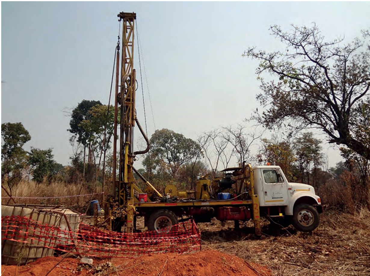
Photo 1: Drill rig on site at Luansobe
