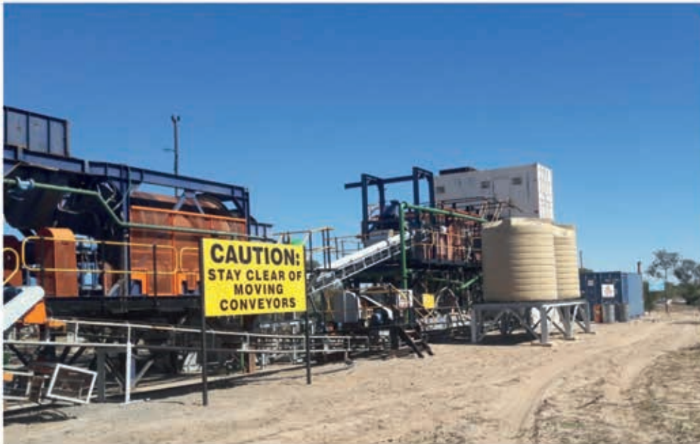
Figure 4: KX36 Bulk sampling plant (photo: Petra Diamonds Ltd)
