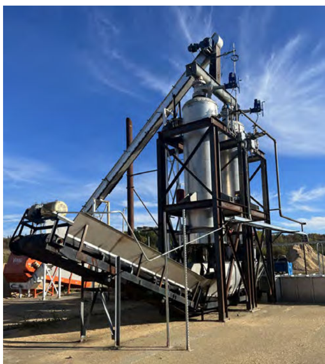
CoalSwitch® reactor - Ashland
