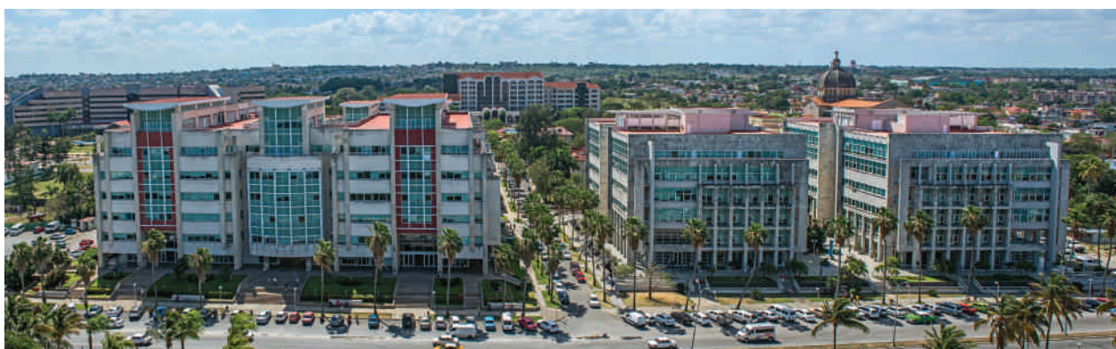
View of the Miramar Trade Center commercial real estate complex from 3 rd Avenue
