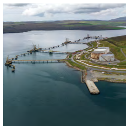
EnQuest operates the Sullom Voe Terminal on Shetland, which will be the focus of the Company's decarbonisation and new energy projects
