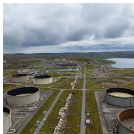
View of Central Avenue Sullom Voe Terminal
