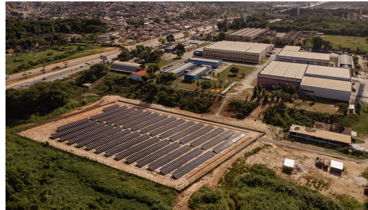
The company's first solar energy plant in Brazil was inaugurated at our Recife plant. A total of 1,580 panels have been installed, which will supply nearly 30% of the location's electricity requirements. It marked another important step towards achieving our ambition of reducing carbon emissions in our own operations by 50% by 2030.
